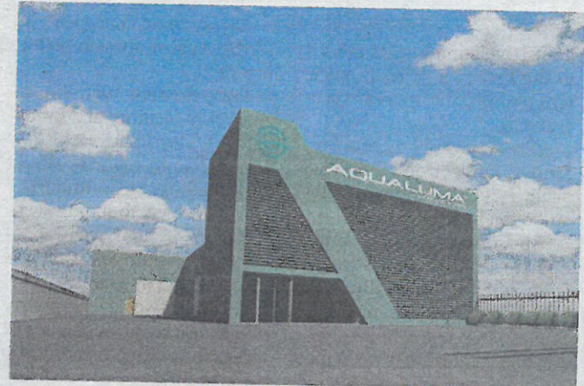
An image of the Aqualuma building taking shape on Siganto Drive.
